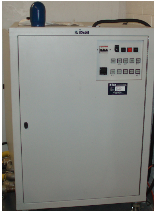
Figure C.1: ISA water skid system.
