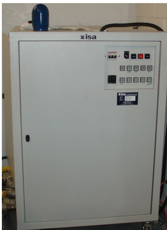
Figure C.1: ISA water skid system.
