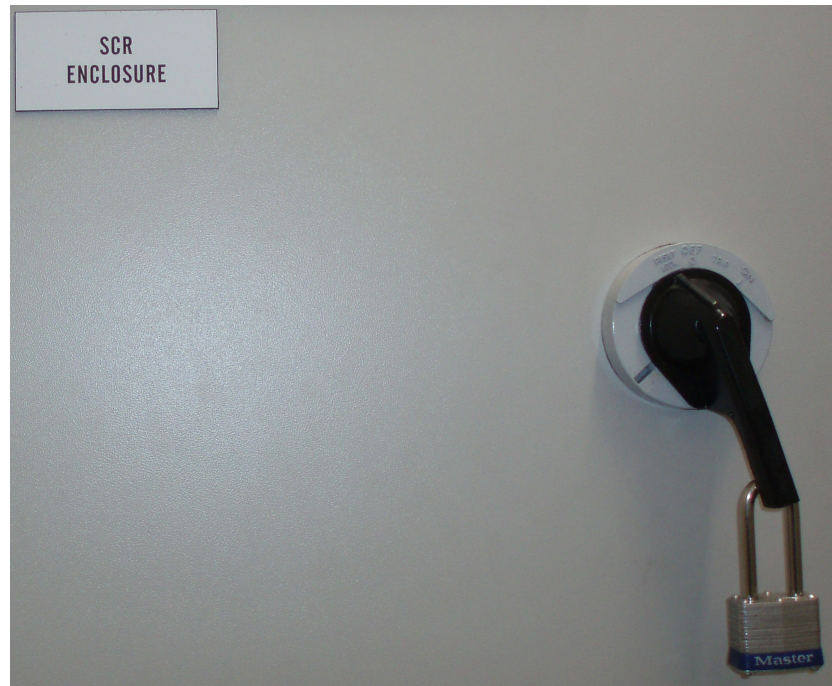
Figure C.2: SCR enclosure and the padlock.
