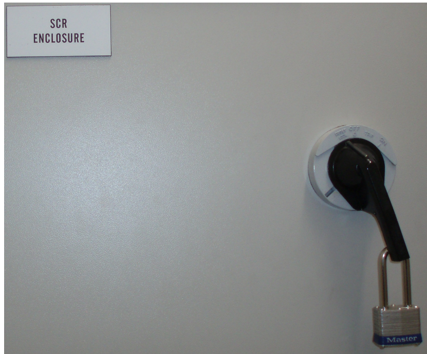
Figure C.2: SCR enclosure and the padlock.
